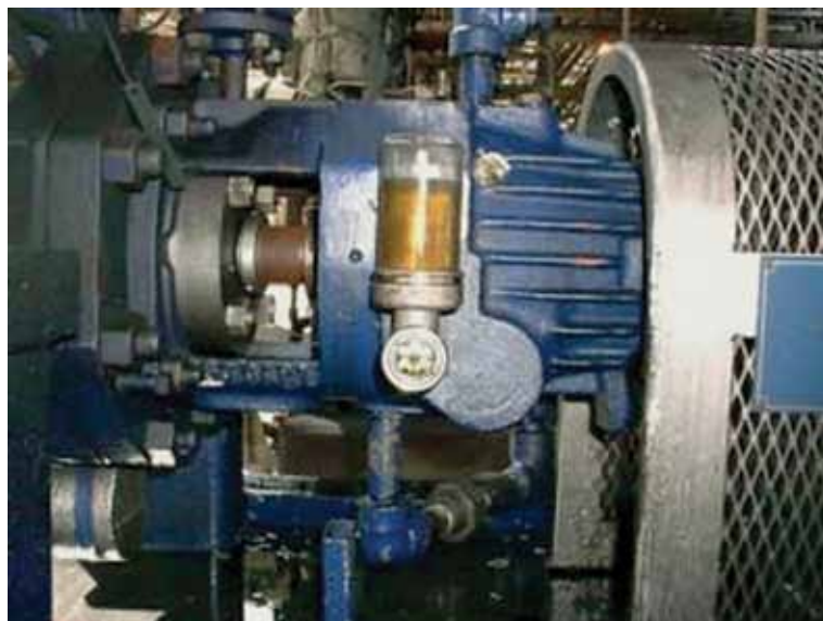
Watchdog Oiler Installation
